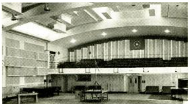
Below: BBC Maida Vale studio one, featuring new acoustical treatment recently applied to walls above and below balcony to improve the reverberation and frequency response of the studio.
